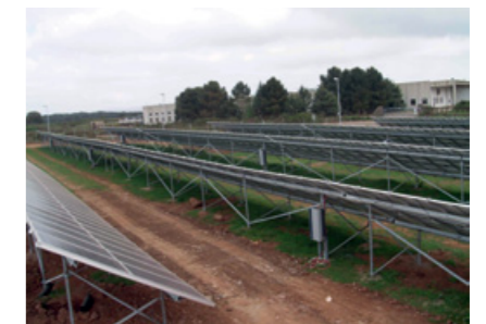
1MWp, ground-mounted installation, commissioning: 2011
