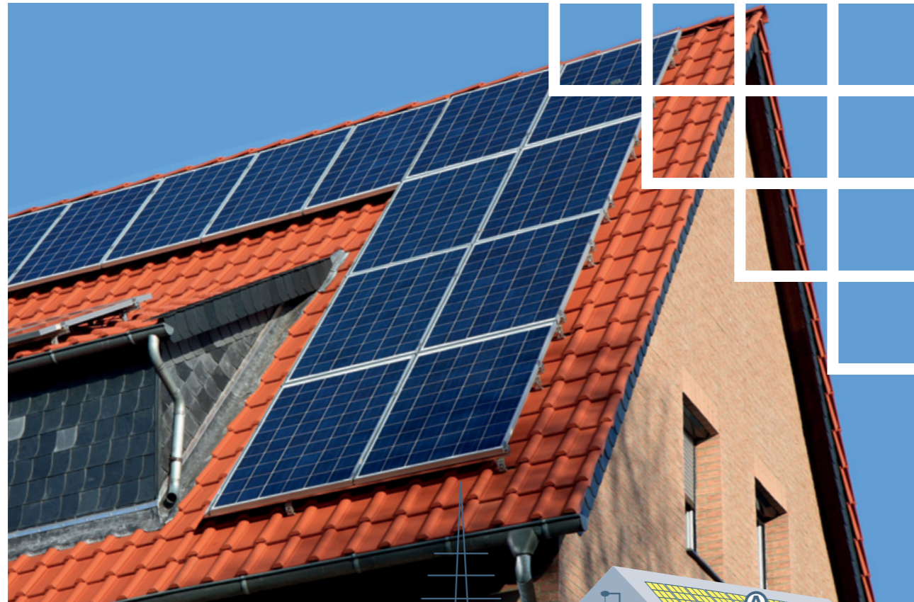
Differently oriented roof surfaces and shading
