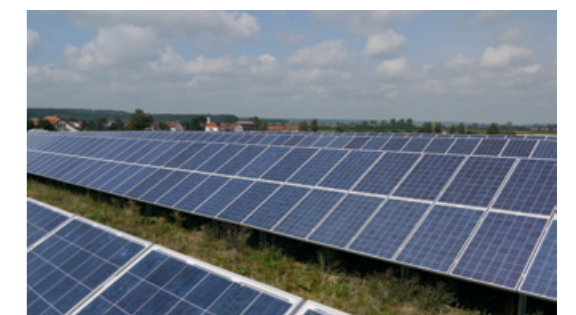
265 kWp, ground-mounted installation, commissioning: 2010
